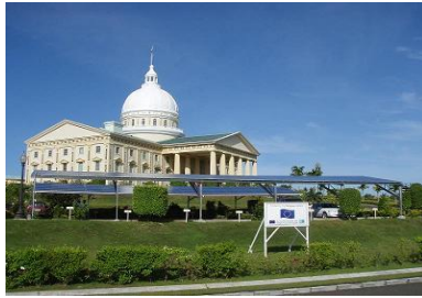
Grid-connected PV system for the Capitol complex –100kW p , Cost: 1,040,000 Euros
