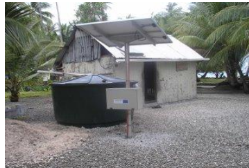
420 Solar Home Systems- 200W p each Cost: 1.35 Million Euros
